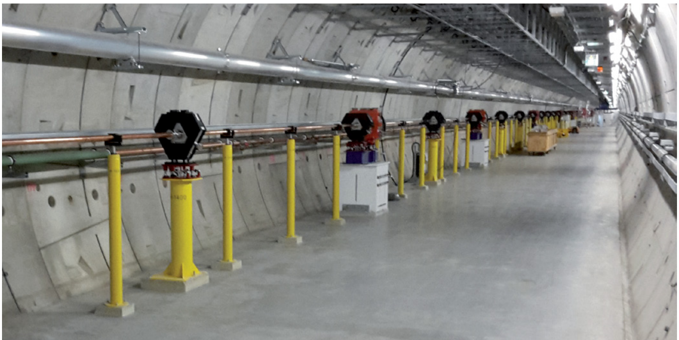
Agilent In-line Ion pumps integrated into a transport beam-line at X-FEL/Desy
